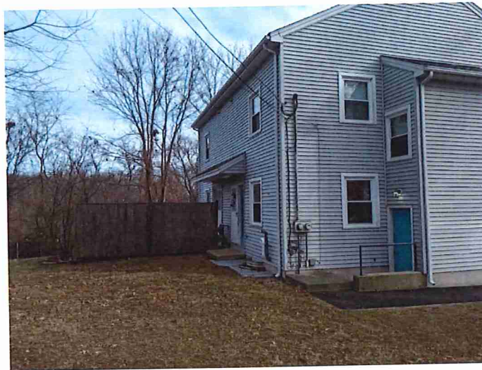
Side and rear elevations (from January 19, 2021 inspection)
