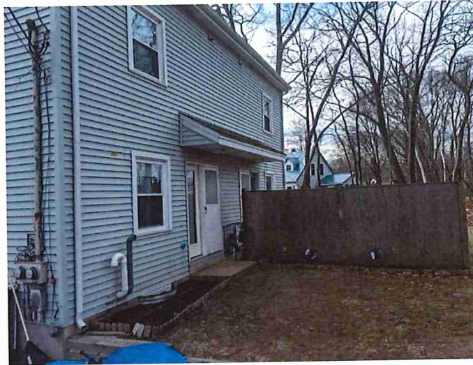
Rear elevation (from January 19, 2021 inspection)
