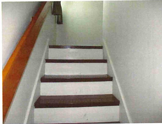
Interior unit staircase
